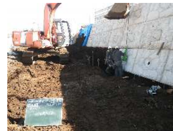
擁壁施工例①
