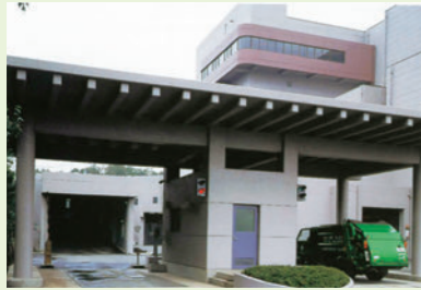
計量棟 Truck scale building
